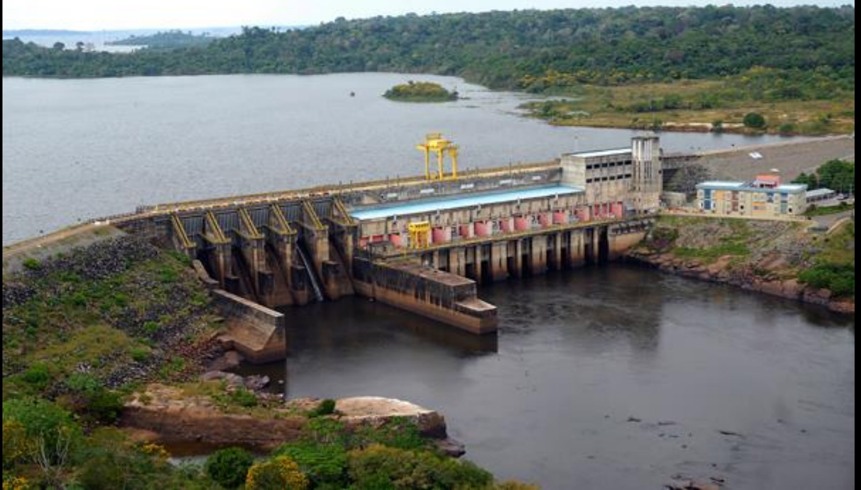
Samuel Hydroelectric Dam, 216 MW, Rondônia, Brasil. Photo: www.irn.org
